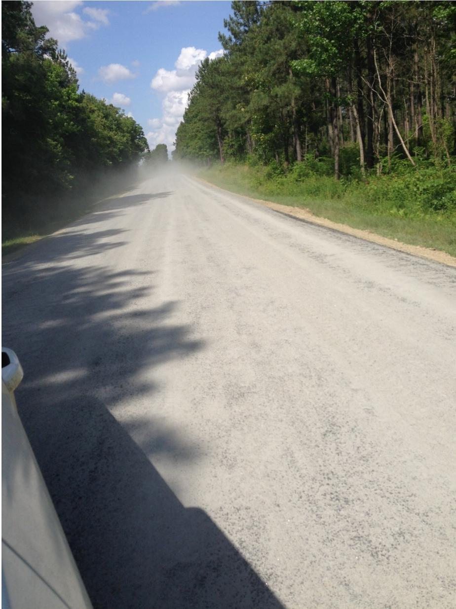
Figure 27. Excessive Aggregate.
