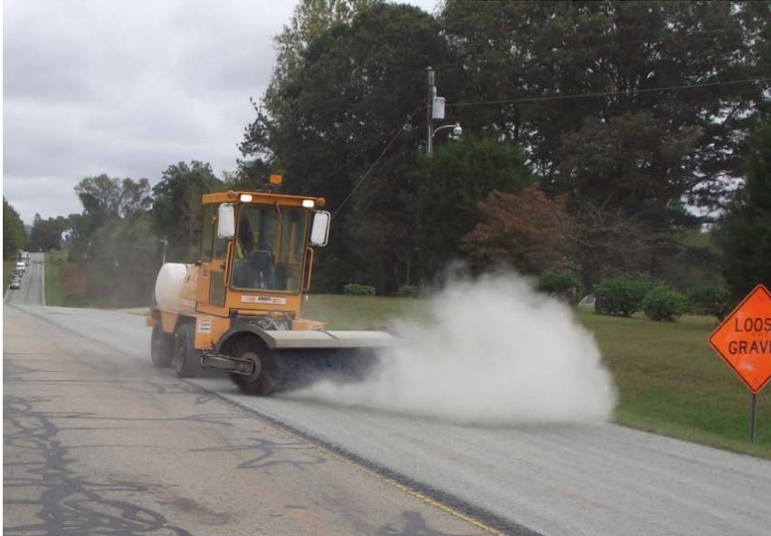
Figure 10. Mechanical broom operation.
