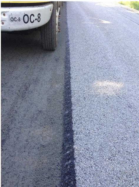
Figure 28. Centerline Tie Strip – Longitudinal Joints.
