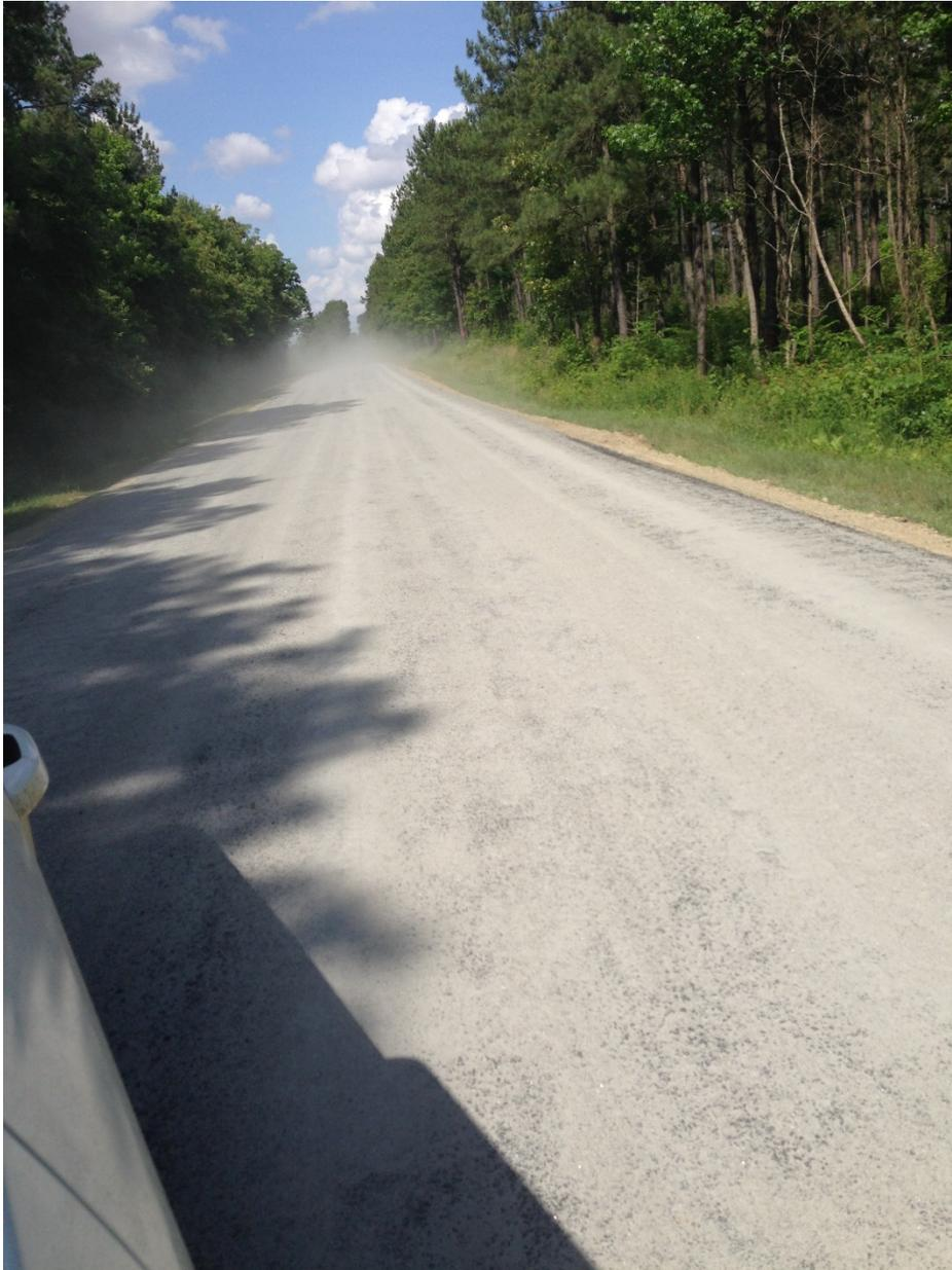
Figure 27. Excessive Aggregate.
