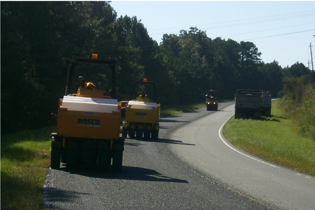
Figure 21. Two pneumatic tire rollers followed by a static steel wheel roller or combination roller.
