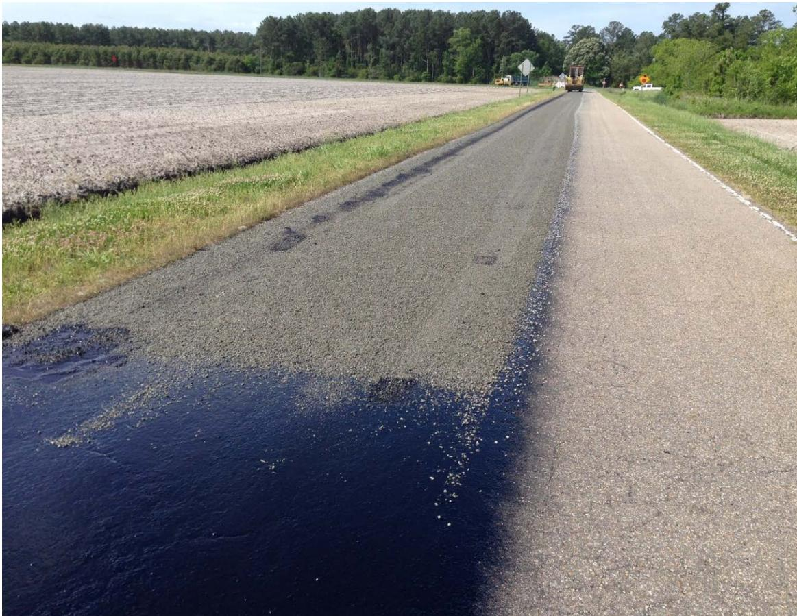
Figure 26. Insufficient Aggregate.
