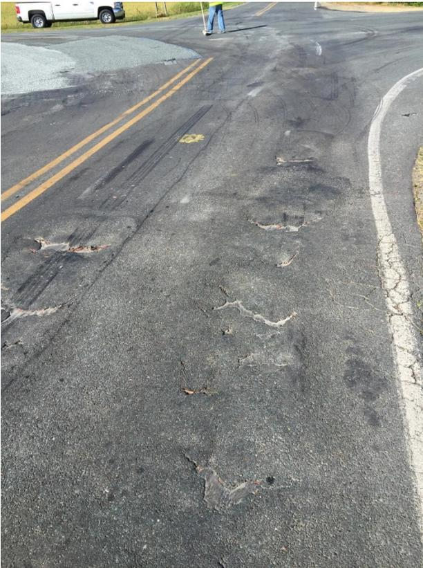
Figure 4. Severe Alligator Cracking.
