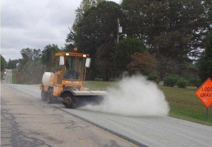
Figure 10. Mechanical broom operation.
