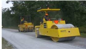
Pneumatic tire roller (in background) being followed by a static steel roller (in foreground)
