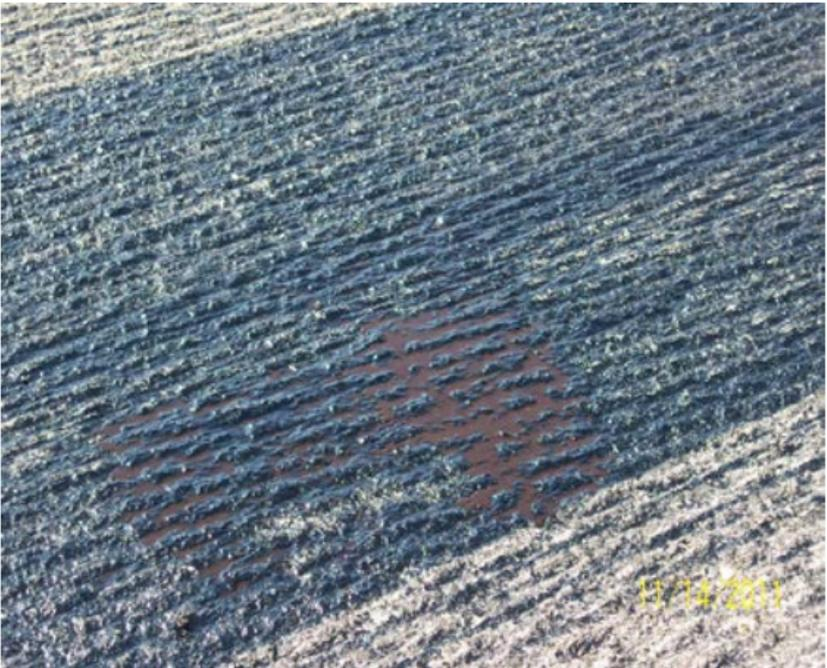
Tack coat will turn from a **brown** color after placement on the surface to a **black** color after it breaks.
