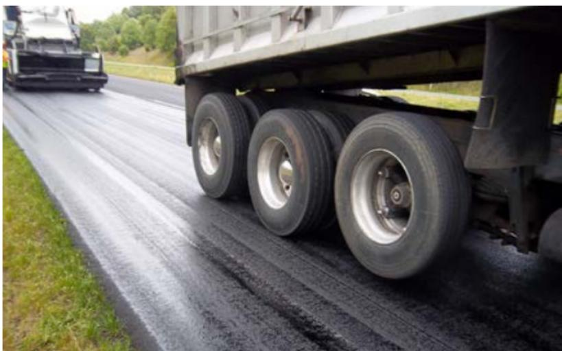
Non-tracking tack coat is a form of tack coat with formulations so that it does not track after it is placed. Contractor is allowed to use non-tracking tack coat as an option.
